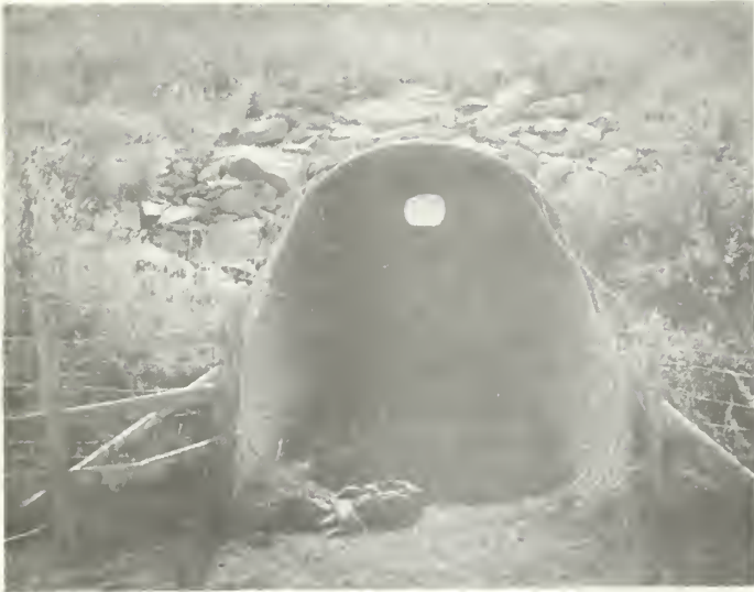
NORTH ENTRANCE; Notice bulge
